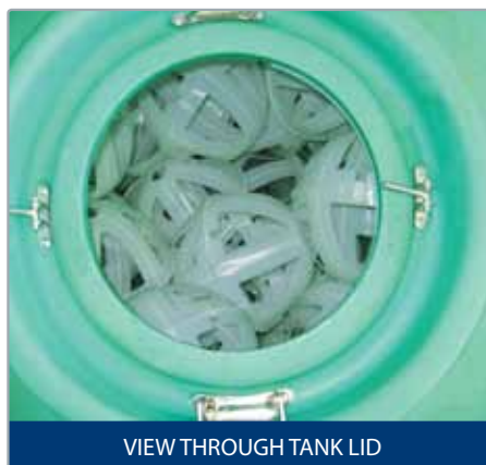
INTERNAL VIEW OF TANK WITH BALL BAFFLES
